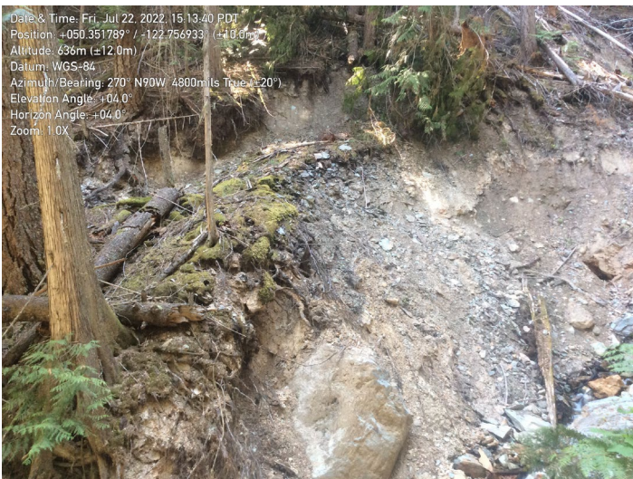
Photo 12. Fresh point source release on right bank sidewall.
