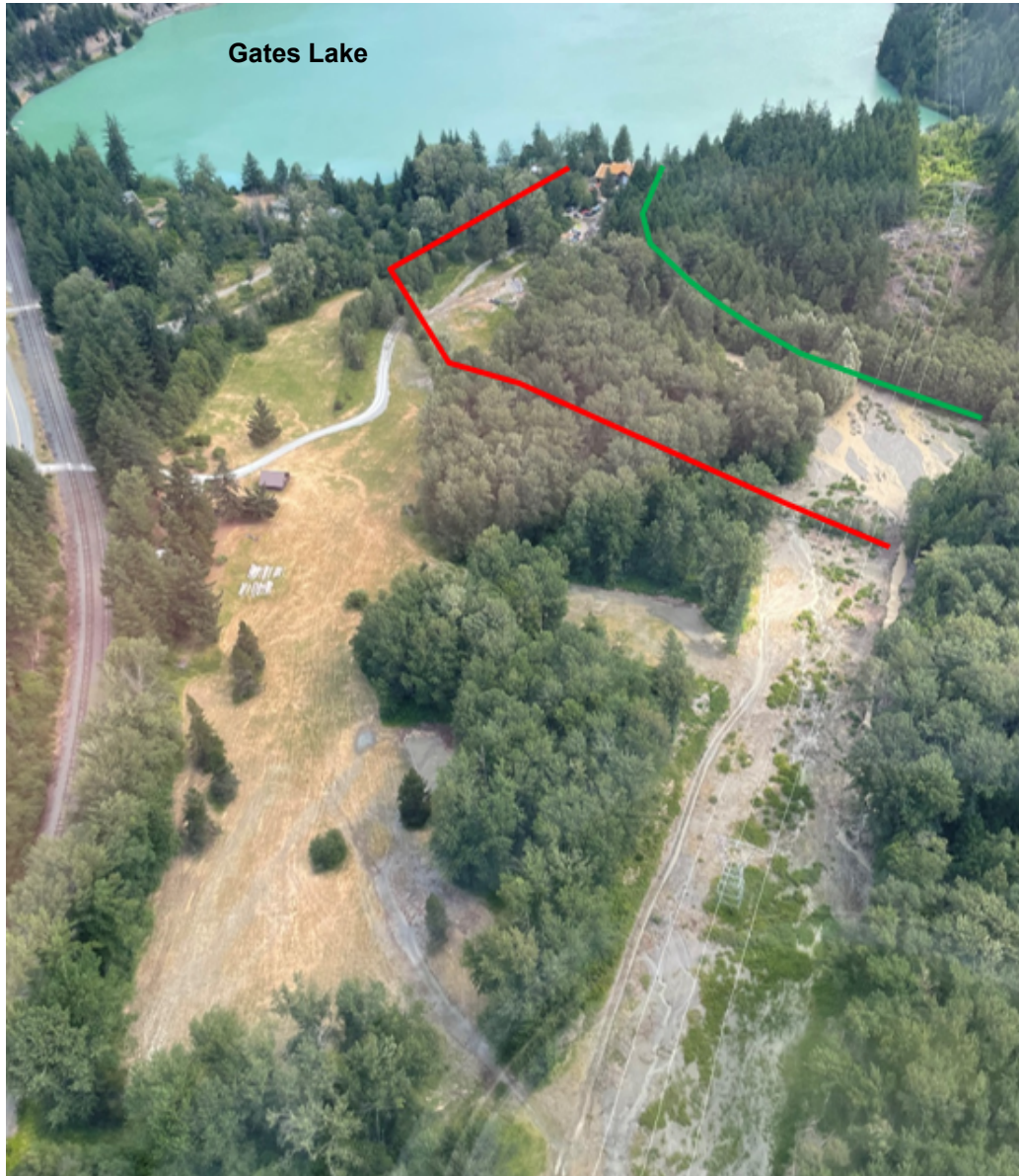
Figure 7 - Post Event Place Creek Flow Conveyed Through Man-Made Drainage Ditches (Red and Green Solid Lines - Stantec, July 24, 2024)
