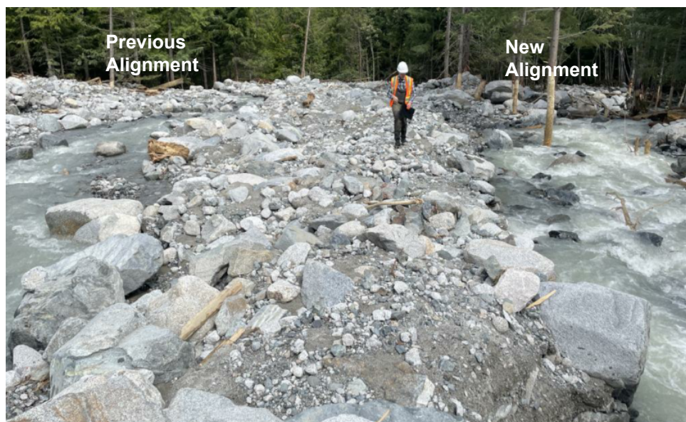
Figure 13 – Looking Downstream At New (Right) and Previous (Left) Place Creek Alignments
