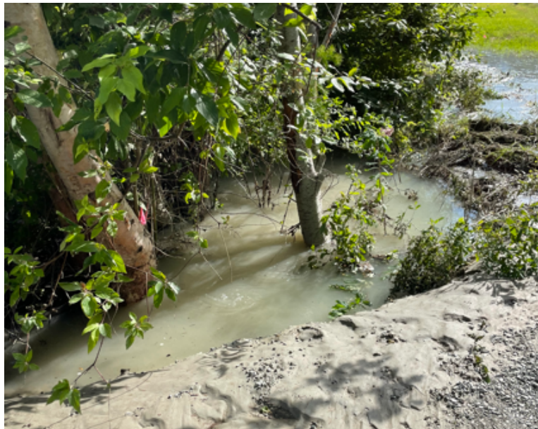
Figure 22 – Overland Flooding Due to Undersized Constructed Ditch Conveying Place Creek Flow
