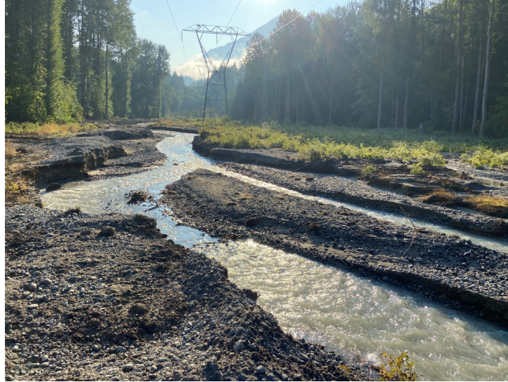
Figure 24 – Overland Flow Along New Place Creek Alignment Through BC Hydro ROW Following Aug 4/5 Rainfall Event.
