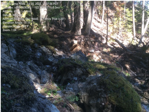
July 20, 2022. Headscarp of main instability. Waypoint 19, Appendix 1.
