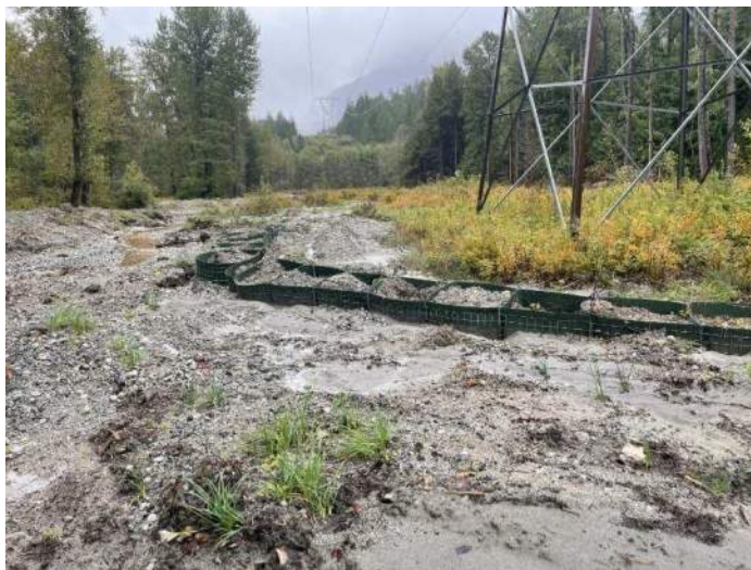
Image 2: BC Hydro tower prior to gabion basket removal (looking east) (2024-09-25)
