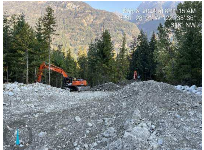
Image 3: 350 and 210 excavators working together to excavate proposed channel, and stockpile materials to build up the proposed embankment (2024-09-06 @ 8:11 AM)
