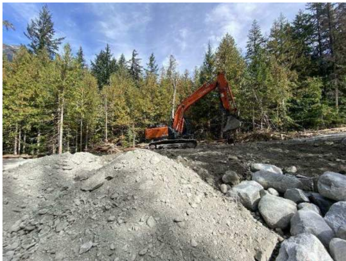
Image 4: 210 excavator working on the embankment downstream of the diversion point. (2024-09-16 @ 1:22 PM)
