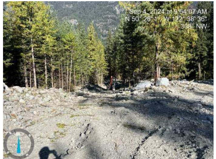
Image 13: 210 excavator continued to excavate the proposed channel (2024-09-04 @ 9:54 AM)
