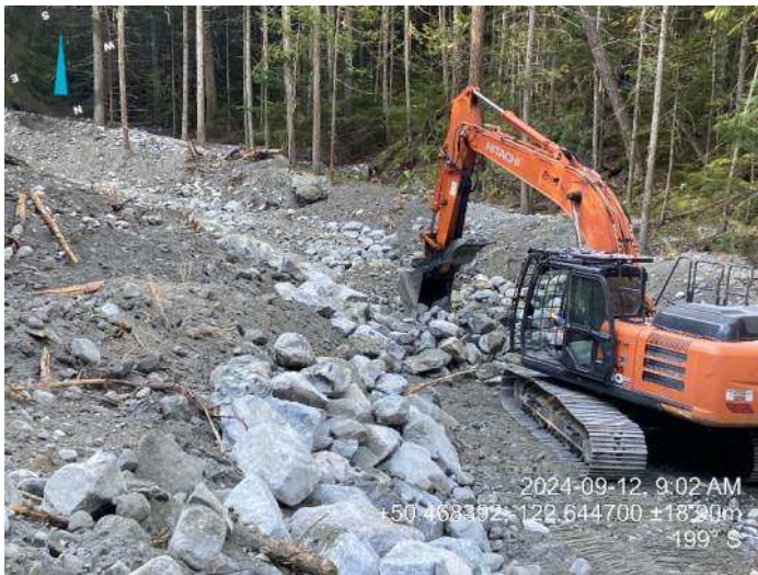
Image 4: 210 excavator adding boulders to channel bed (2024-09-12 @ 9:02 AM)
