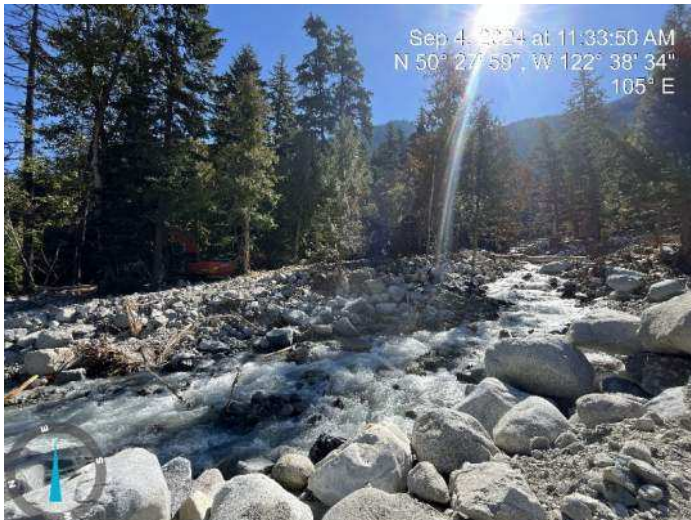
Image 16: 350 excavator building up the proposed embankment (2024-09-04 @ 11:33 AM)
