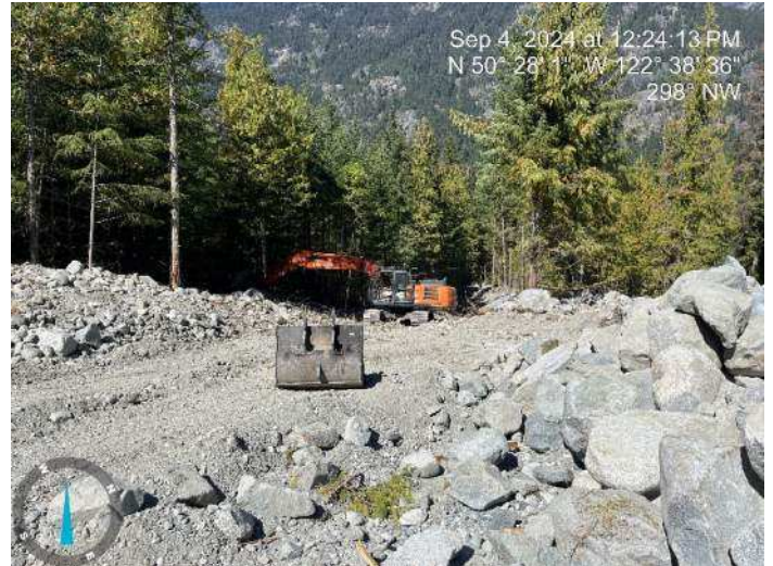
Image 19: 210 excavator continued to excavate the proposed channel (2024-09-04 @ 12:24 PM)
