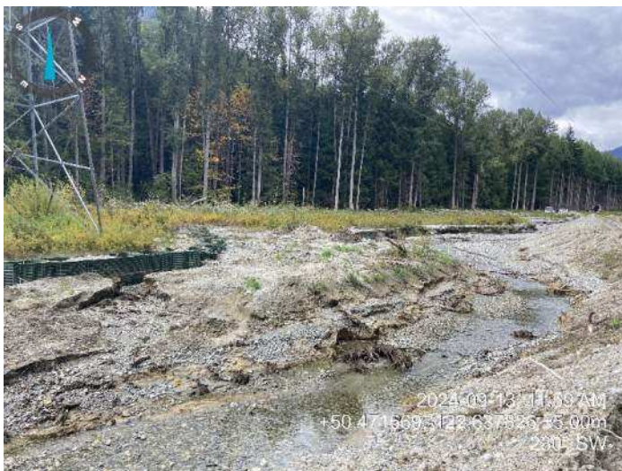
Image 10: ditch constructed as part of the early emergency works (2024-09-13 @ 11:59 AM)
