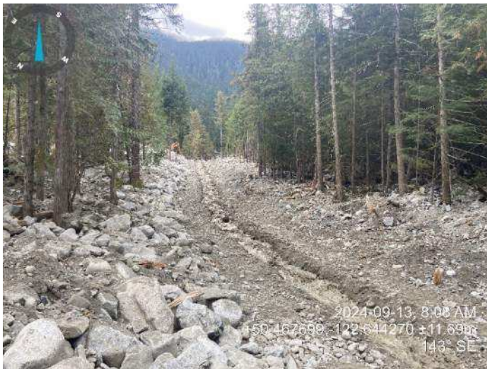
Image 4: water in Place Creek flowing through the notch in the centre of the reestablished channel (2024-09-13 @ 8:08 AM)
