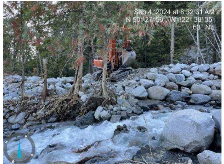
Image 7: 350 excavator continued to reinforce the toe of the proposed embankment (2024-09-04 @ 8:32 AM)
