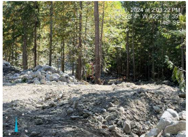
Image 13: 250 excavator continued to excavate the proposed channel (2024-09-03 @ 2:03 PM)
