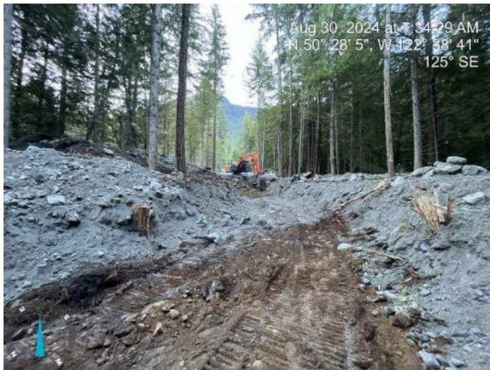
Image 4: 250 excavator continued to excavate the proposed channel (2024-08-30 7:34 AM)
