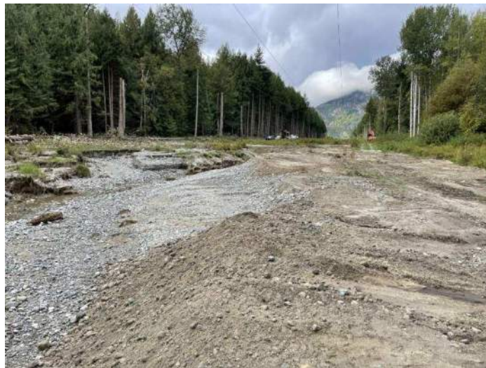
Image 4: Emergency berm removed with material placed over access road (looking west) (2024-09-23)
