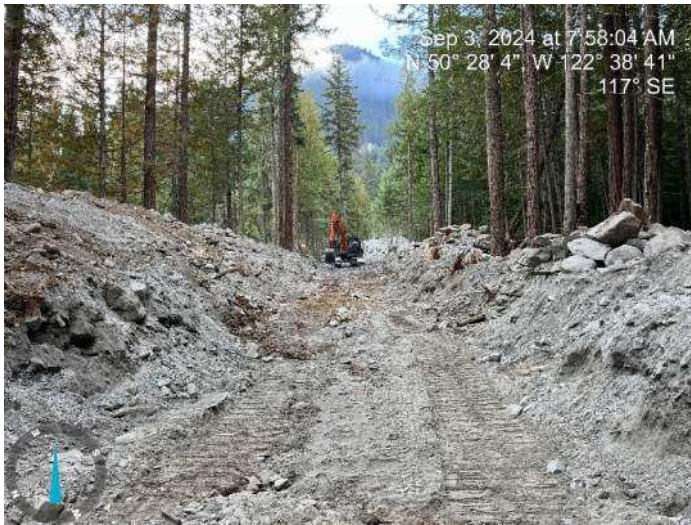
Image 2: 250 excavator continued to excavate the proposed channel (2024-09-03 7:58 AM)
