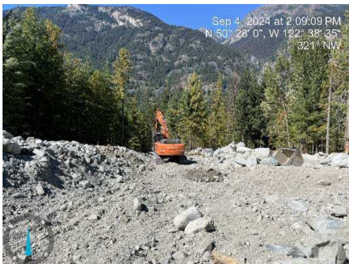
Image 20: 210 excavator continued to excavate the proposed channel (2024-09-04 @ 2:09 PM)
