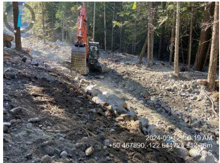
Image 5: 210 excavator adding boulders to channel bed (2024-09-12 @ 10:19 AM)
