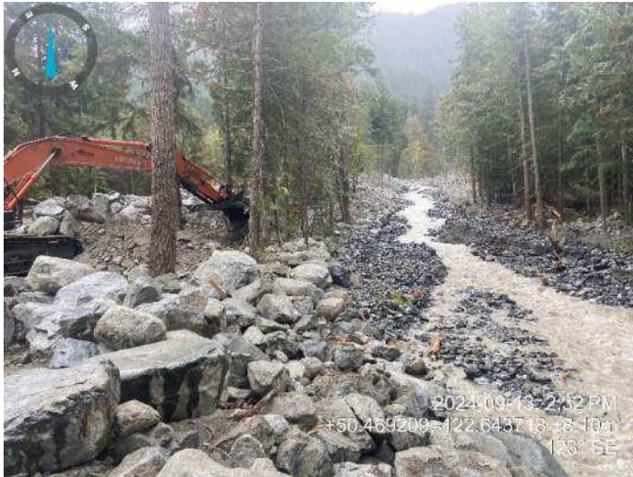
Image 10: 210 excavator adding boulders to the channel bank (2024-09-13 @ 2:32 PM)
