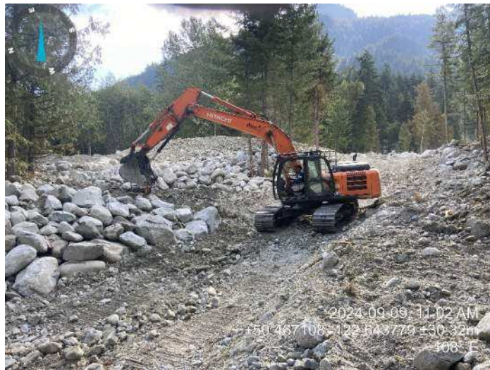
Image 5: 210 excavator armoring the east bank of the channel and embankment (2024-09-09 11:02 AM)
