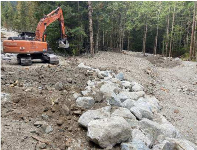
Image 4: 210 excavator embedding boulders to protect toe of embankment from erosion (2024-09-10 8:31 AM)
