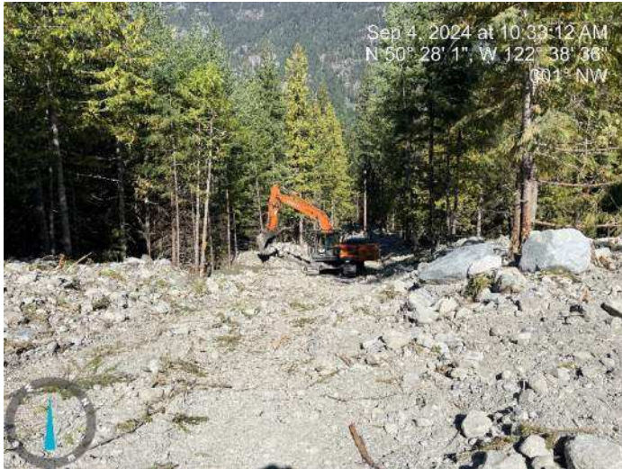
Image 14: 210 excavator continued to excavate the proposed channel (2024-09-04 @ 10:33 AM)
