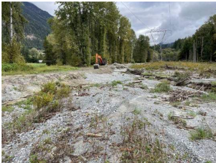
Image 3: Emergency berm removed with material infilling emergency ditch (looking east) (2024-09-23)
