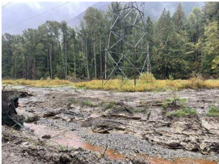
Image 3: BC Hydro tower following removal of gabion baskets (looking south) (2024-09-25)
