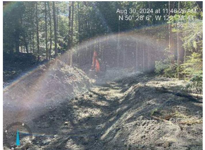
Image 13: 250 excavator continued to excavate the proposed channel (2024-08-30 @ 11:46 AM)
