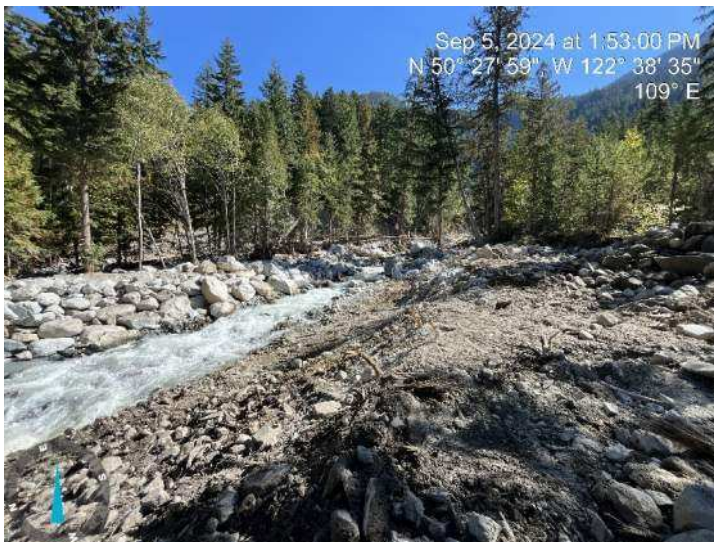
Image 22: Existing channel condition at time of departure (2024-09-05 @ 1:53 PM)
