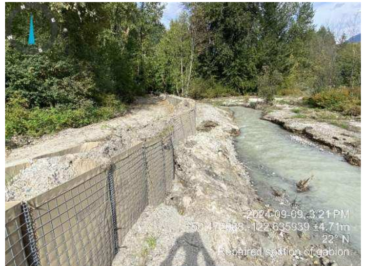
Image 9: Looking downstream at the previously repaired section of gabion bags (2024-09-09 @ 3:21 PM)
