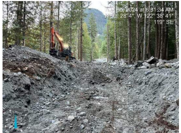
Image 3: 250 excavator excavating the proposed channel (2024-08-30 @ 6:31 AM)
