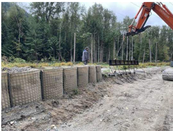
Image 5: Removing emergency gabion baskets (2024-09-23)
