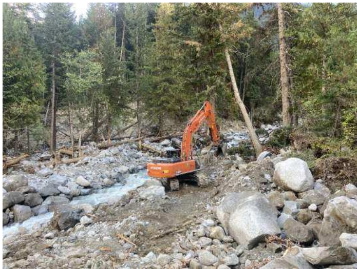
Image 4: 350 excavator armoring east bank (2024-09-09 10:18 AM)
