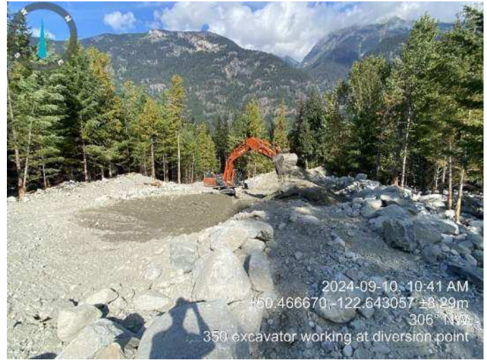
Image 3: 350 excavators moving large boulder to prevent flow from impinging on the embankment (2024-09-10 @ 10:41 AM)
