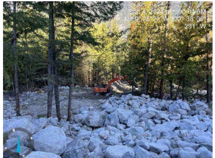
Image 9: 210 excavator continued to excavate the proposed channel (2024-09-04 @ 9:00 AM)
