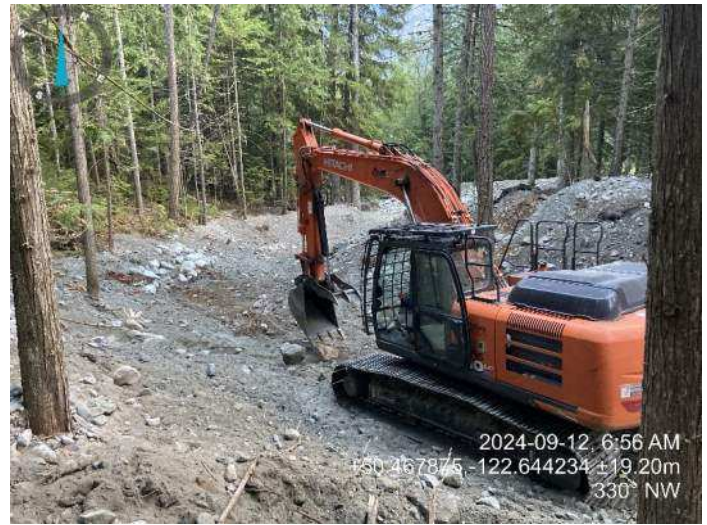
Image 3: 210 excavator adding boulders to channel bed (2024-09-12 @ 6:56 AM)
