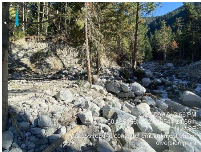
Image 3: access route to construct embankment upstream of diversion point (2024-09-16 @ 3:56 PM)
