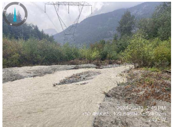
Image 11: Flow in the reestablished channel beneath the hydro corridor after diverting flow (2024-09-13 @ 2:49 PM)
