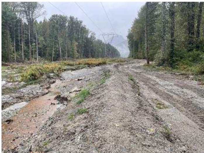
Image 5: Portion of emergency berm left in place (looking west) (2024-09-25)
