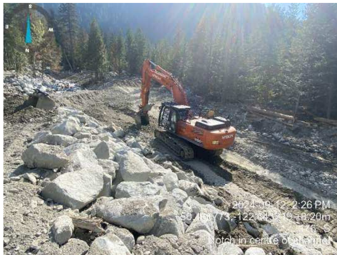
Image 7: 350 excavator cutting a notch in the center of the channel (2024-09-12 @ 2:26 PM)
