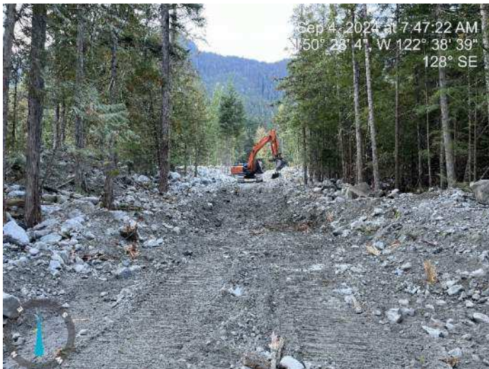
Image 4: 210 excavator continued to excavate the proposed channel (2024-09-04 7:47 AM)
