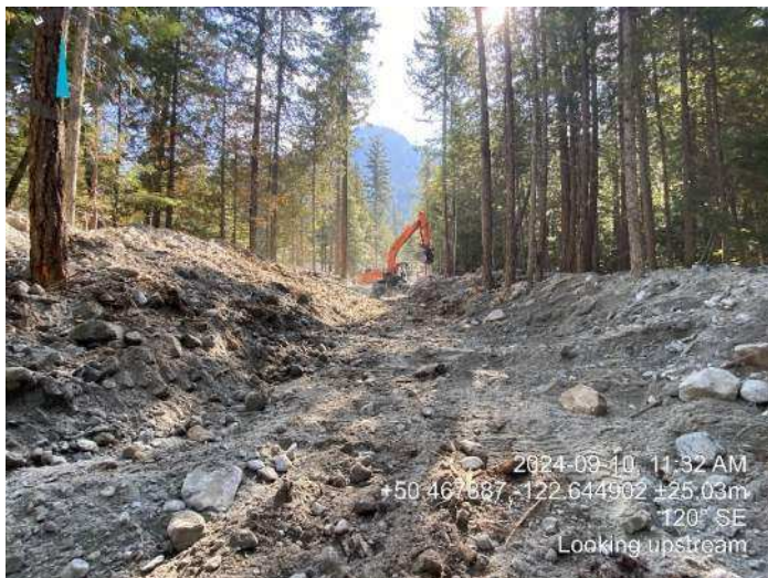
Image 6: 210 excavator regrading channel banks (2024-09-10 @ 11:32 AM)
