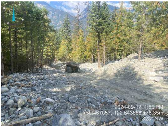
Image 6: rock truck hauling material for embankment (2024-09-12 @ 1:55 PM)
