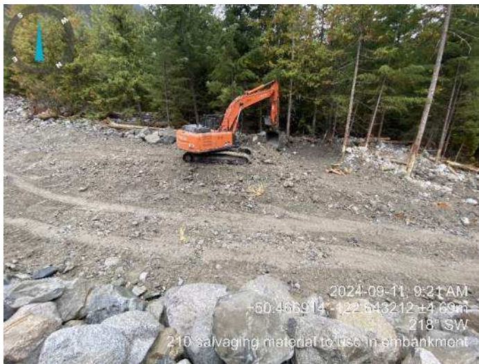
Image 3: 210 excavators moving material to be used on embankment (2024-09-11 @ 9:21 AM)
