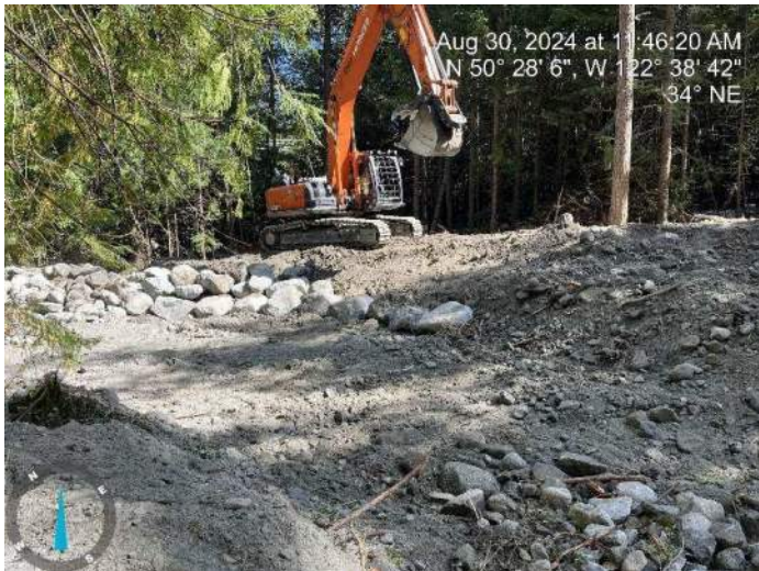
Image 12: 350 excavator placing riprap along the right channel bank looking downstream (2024-08-30 @ 11:46 AM)
