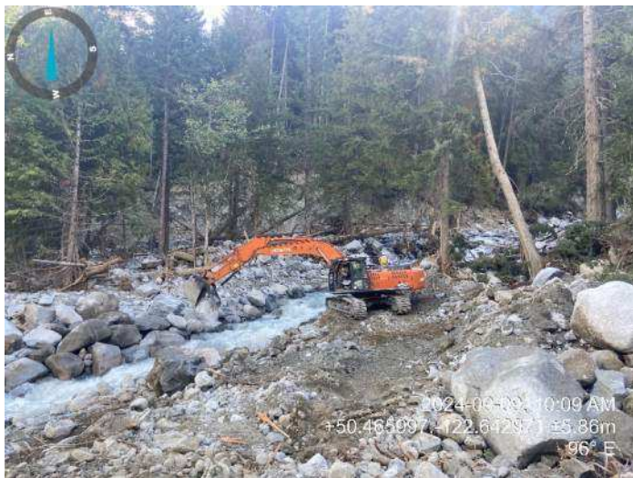
Image 2: 350 excavator armoring east channel bank above diversion point (2024-09-09 10:09 AM)
