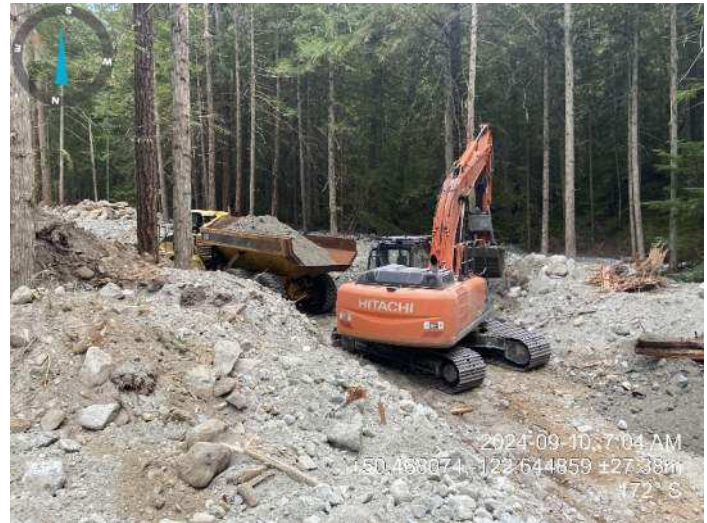
Image 5: 210 excavator regrading channel banks (2024-09-10 7:04 AM)
