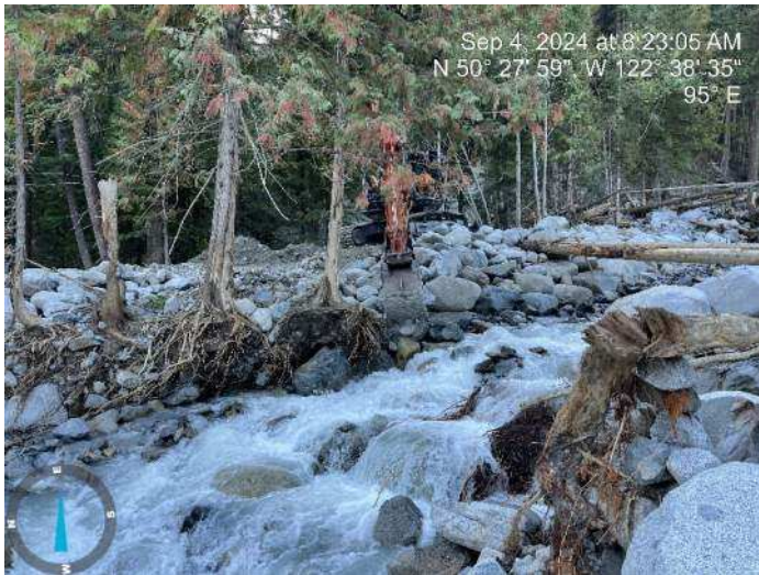
Image 6: 350 excavator continued to reinforce the toe of the proposed embankment (2024-09-04 @ 8:23 AM)
