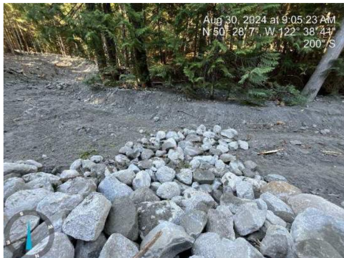
Image 9: Riprap placed along the right channel bank looking downstream (2024-08-30 @ 9:05 AM)
