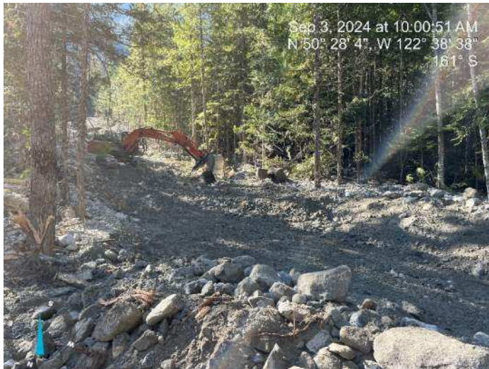
Image 6: 250 excavator continued to excavate the proposed channel (2024-09-03 @ 10:00 AM)
