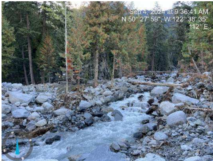
Image 10: Riprap placed on the toe of the proposed embankment along the left bank (looking upstream) of the existing Place Creek channel (2024-09-04 @ 9:36 AM)
