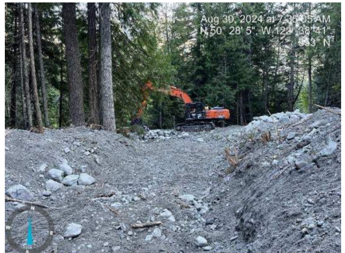
Image 5: 350 excavator placing riprap along the right channel bank looking downstream (2024-08-30 @ 7:35 AM)
