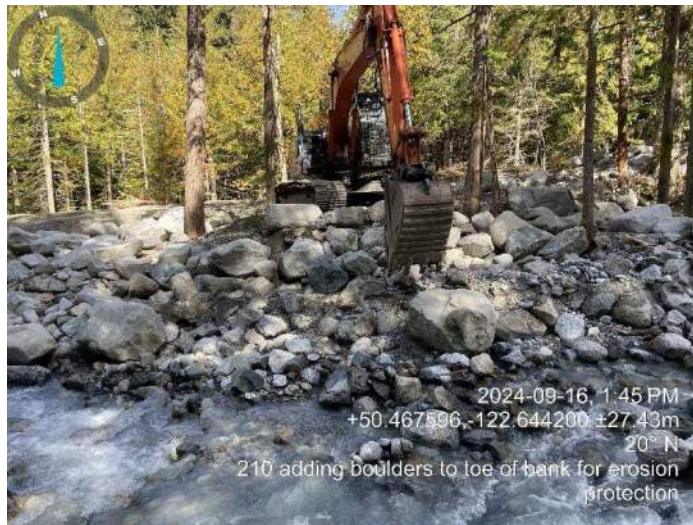
Image 5: 210 excavator adding boulders to the channel bank (2024-09-16 @ 1:45 PM)
