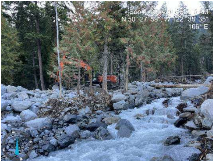
Image 8: 350 excavator continued to reinforce the toe of the proposed embankment (2024-09-04 @ 8:52 AM)
