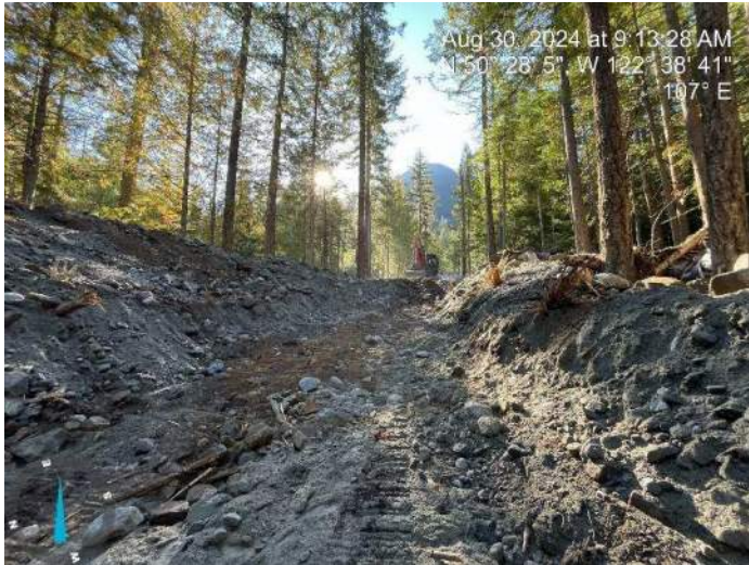
Image 10: 250 excavator continued to excavate the proposed channel (2024-08-30 @ 9:13 AM)
