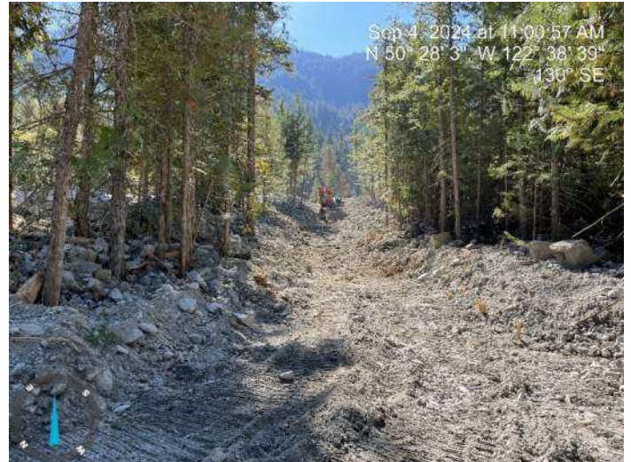
Image 15: 210 excavator continued to excavate the proposed channel (2024-09-04 @ 11:00 AM)
