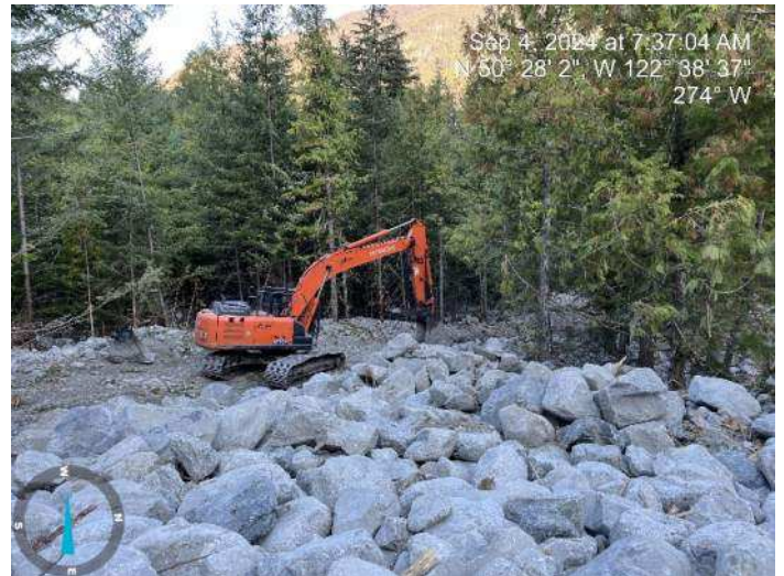
Image 3: 210 excavator continued to excavate the proposed channel (2024-09-04 @ 7:37 AM)
