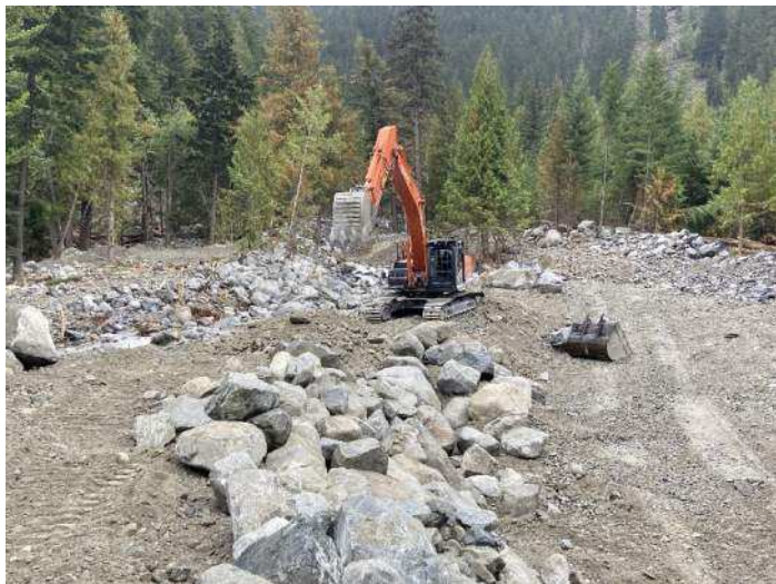
Image 4: 350 excavator working on the diversion point (2024-09-11 12:47 AM)
