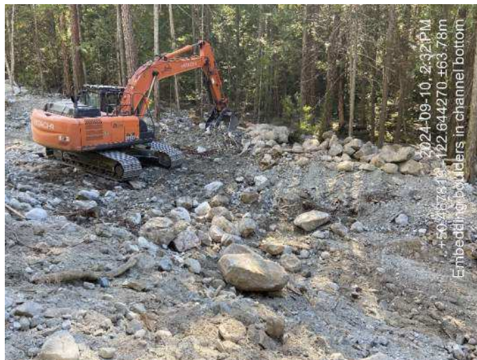
Image 7: 210 excavator embedding boulders on bottom of channel. (2024-09-10 @ 2:32 PM)
