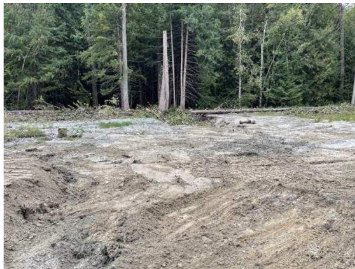
Image 2: upstream extent of emergency ditch that extended across BC Hydro ROW tying into flood channel plugged with emergency bank material (looking south) (2024-09-23)
