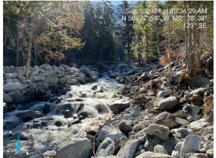
Image 15: Condition of right bank of the existing channel at 10:34 AM on 2024-09-05
