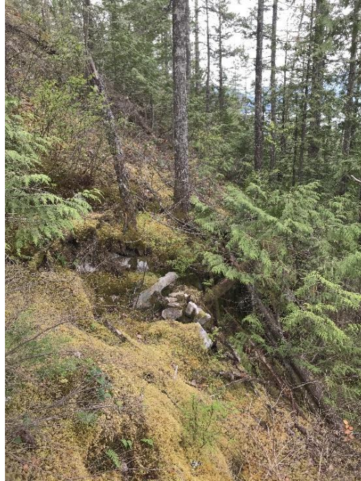
PHOTO 19: View of Upper Benchlands area showing shallow sloughing (indicated by hummocky ground and tilted trees) in overburden veneer over bedrock. (Photo taken by Thurber in May 2019).
